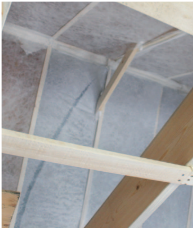
Figure 6. When filling rafter cavities, the usual insertion point is just above the top plate (above). The natural curvature of the longer hose required tends to direct the flow of insulation to one side of the cavity, so filling it uniformly requires a second pass with the curve facing the other way. The hose is visible behind the netting in the photo at right.
