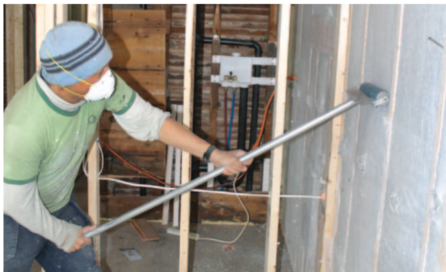
Figure 5. Filled cavities are compacted with an aluminum roller to avoid bulging drywall. A quick pass of the hand is enough to confirm that the insulation lies flush with the framing.
