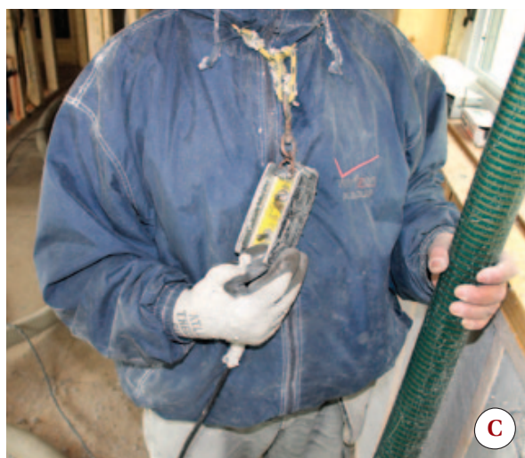
Figure 4. Wall cavities are filled first from the bottom to the midpoint of the wall (A), then from the top back to the middle (B). After a cavity is filled, the operator uses a remote control (C) to momentarily turn off the blower, then quickly inserts the hose into the next cavity before switching it on again.
